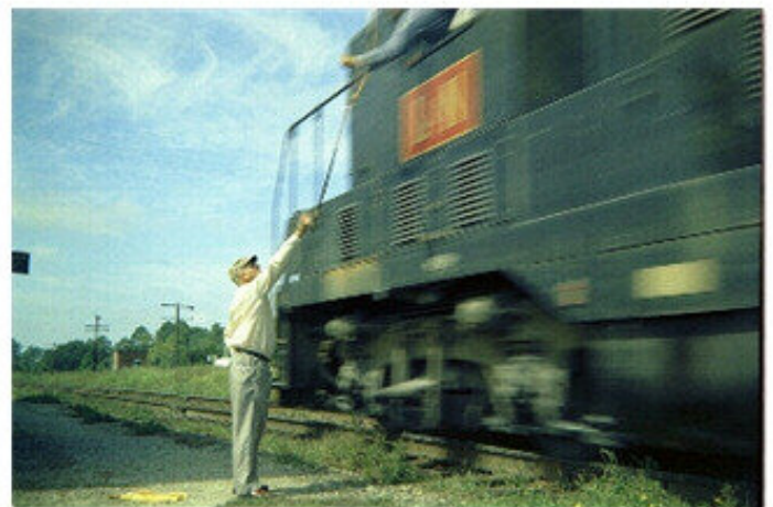
Agent-Operator Robert L. Williams, Saint Elmo, Ala., hoops a message to the crew of Train No. 43 on September 25, 1962. Installation of CTC encompassed his station in 1960, and the train order signal was removed. Thereafter, crews' receipt of necessary messages was taken via Clearance Form A, hooped by the operator using a yellow flag as a signal. Flag was dropped on ground after use and may be seen behind him.
