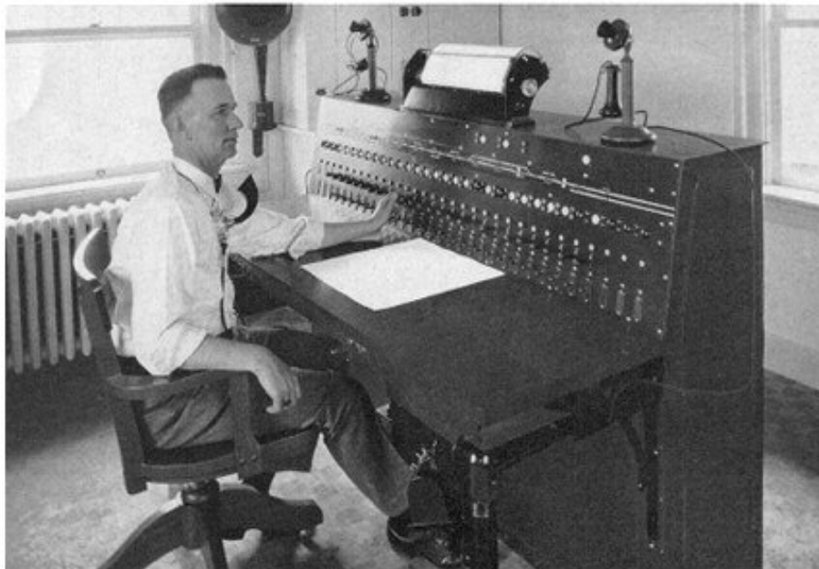
GRS Control Machine of the Stanley to Berwick, Ohio, CTC installation on the NYC
